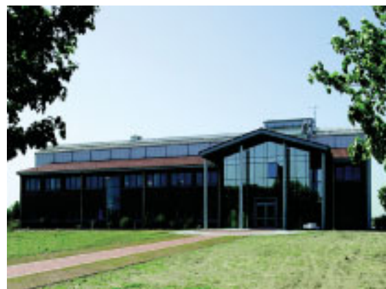
The Albert Einstein Building, the new Optics Building of PTB.
