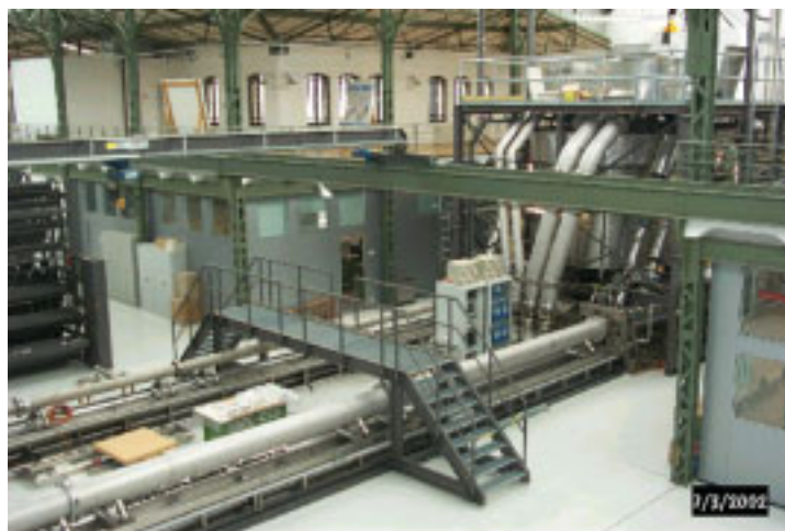
The volume flow measuring facility at the historical Hermann von Helmholtz Building in Berlin with 25 m long measuring sections (nominal diameter: 80 mm and 400 mm) and weighing container (volume: 20 m 3 )
