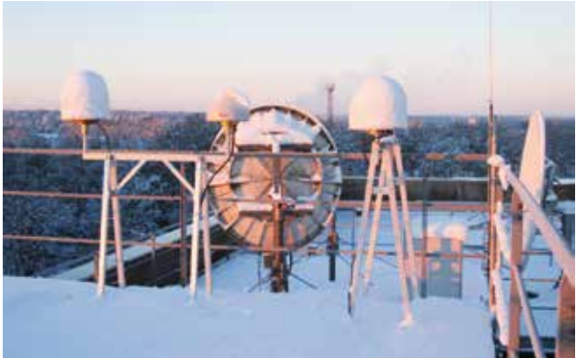
Three antennas for the reception of signals from navigation satellites and two antennas for time comparisons via telecommunications satellites on the roof of the Meitner Building at PTB
