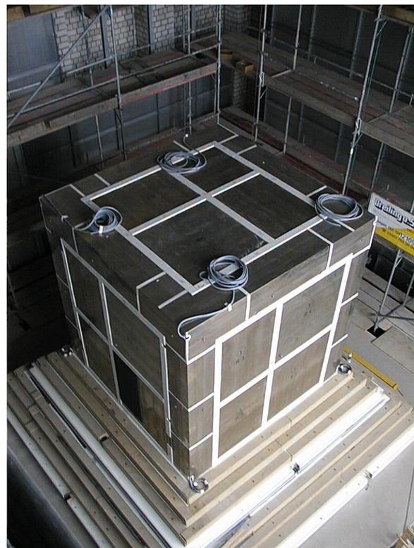
Figure 5: Photograph of the magnetic shield under construction, view on the top, the right wall and the rear wall of the inner cube with the first MUMETALL shell.
