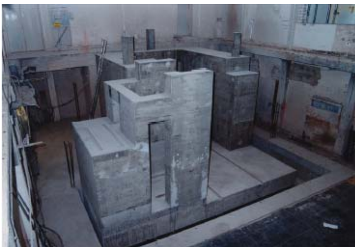
Figure 5. Balance foundation ("raw conditions") with vibration isolation system (right-hand side: location of the vibration isolators)
