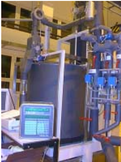
Picture 6: Weighing system 3
